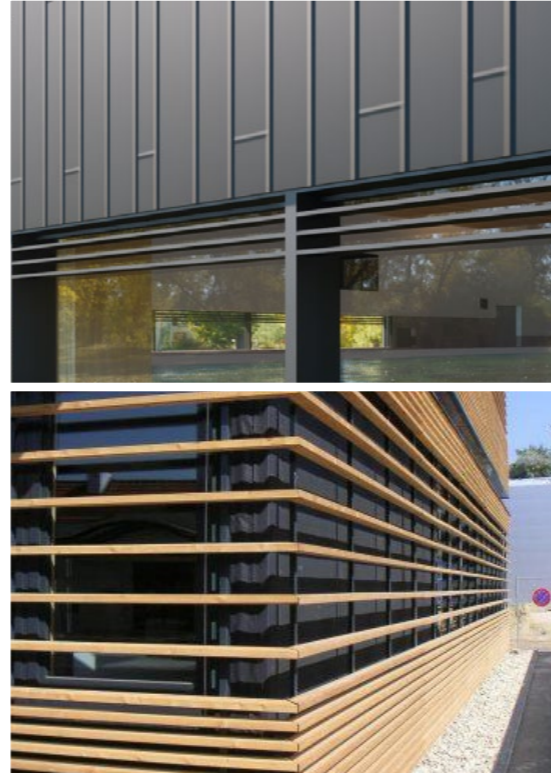
③ Zonwering. Aluminium en houten lamellen.
